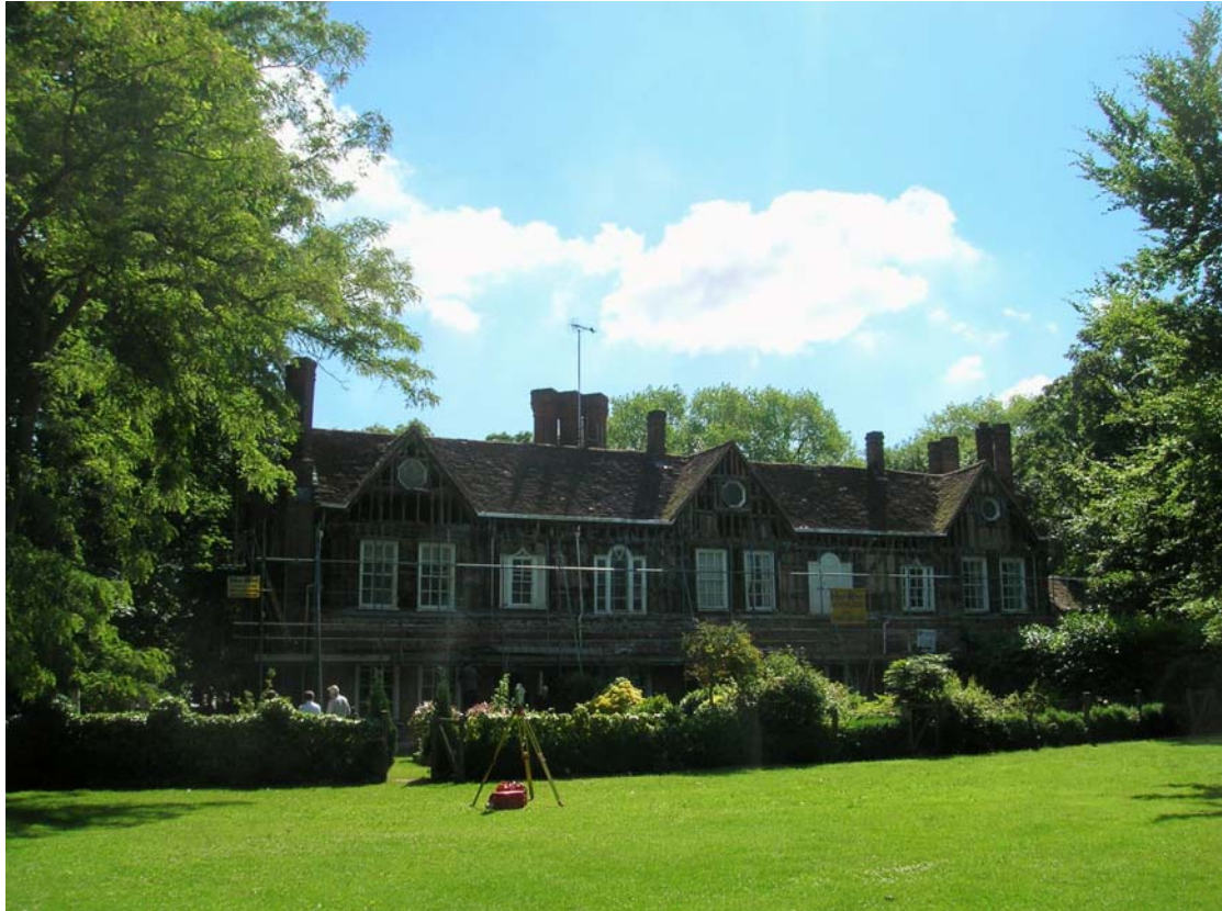
Recording the period timber frame during the phase two work
