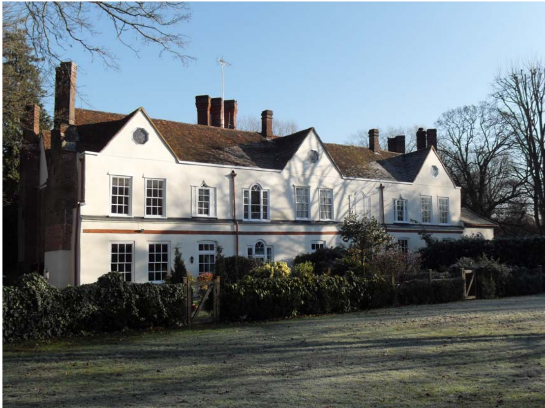
Completion of phase two conservation work
