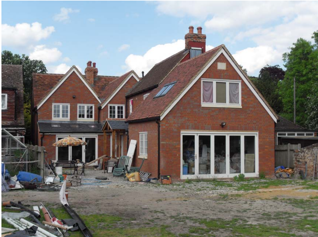
Rear extensions nearing completion
