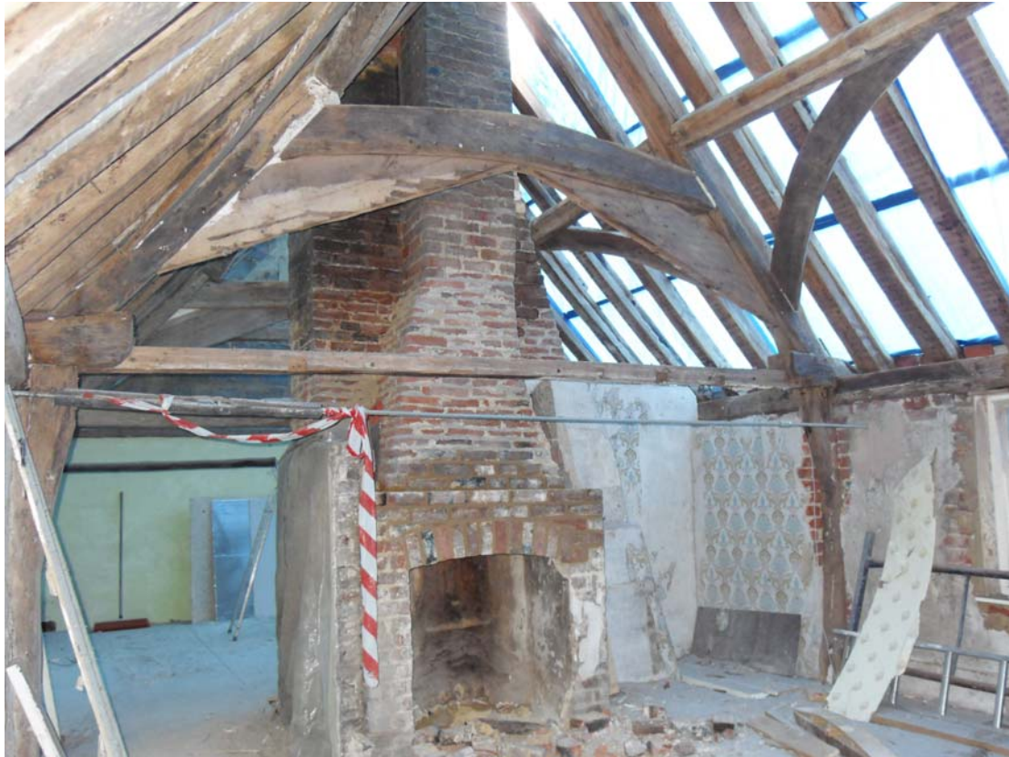
Remaining period timber framed roof structure
