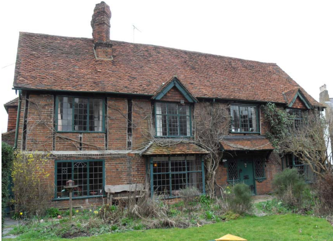
Front elevation before conservation work
