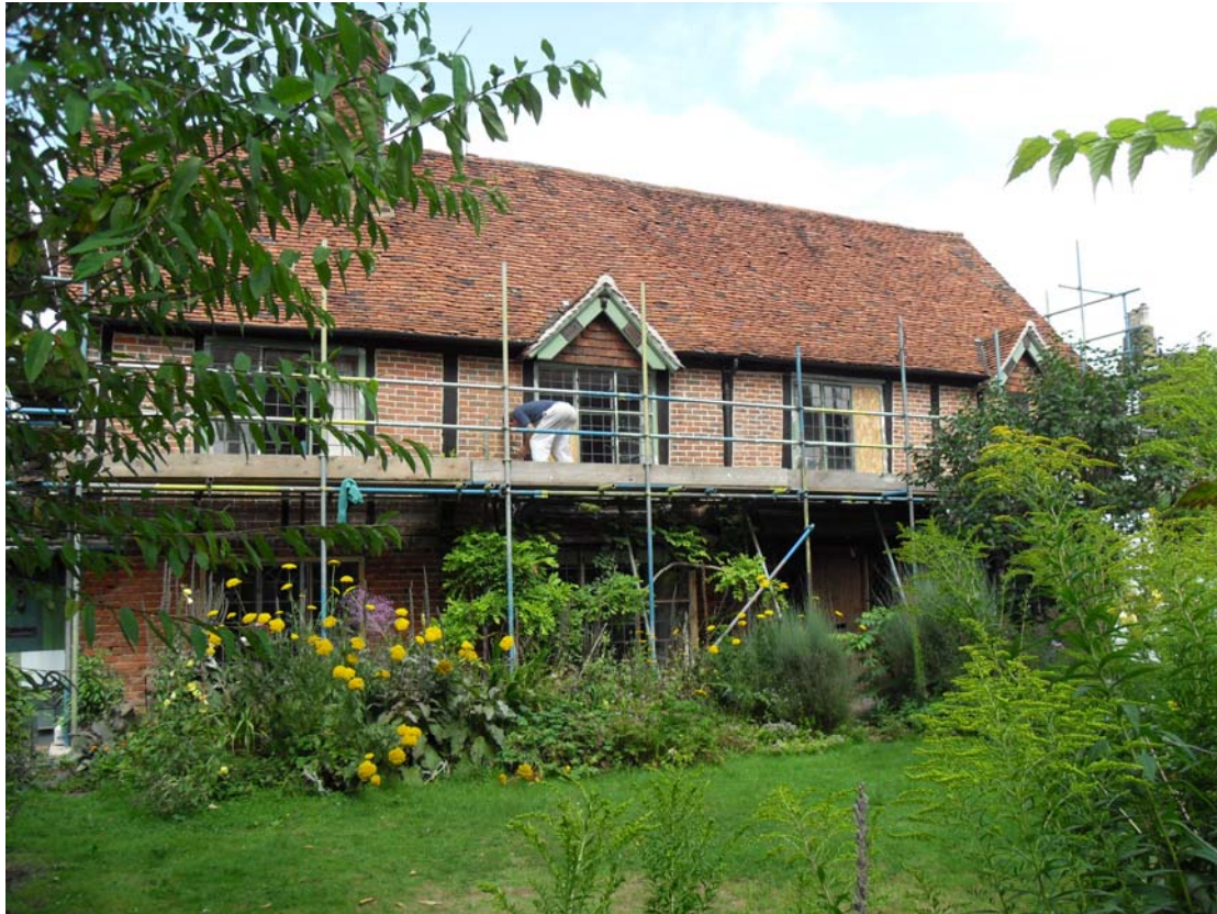
Front elevation repairs in progress
