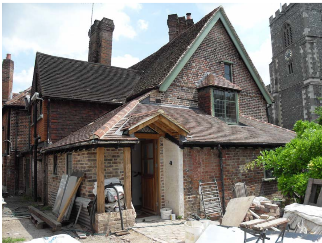
Alterations to the kitchen and utility area nearing completion
